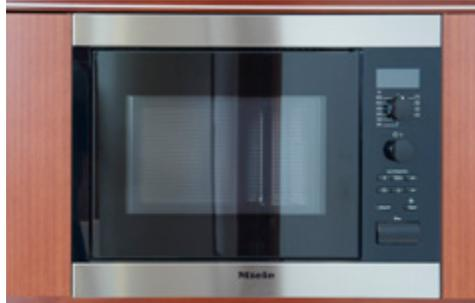
Flush installed microwave in galley
